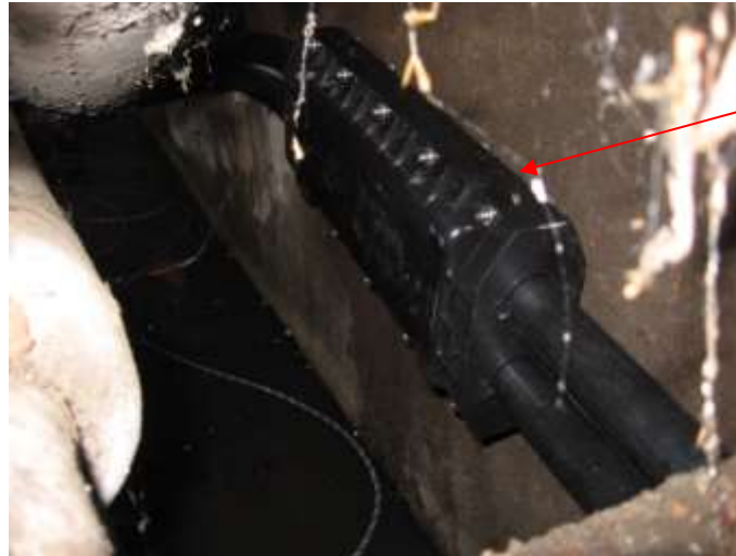
Figure 7 – Typical Installed Multi Subduct joiner
